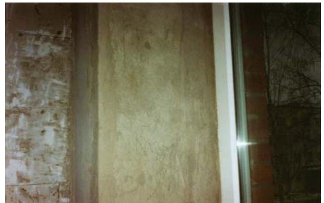
б) A multilayered external wall with an internal layer from porous monolithic concrete
